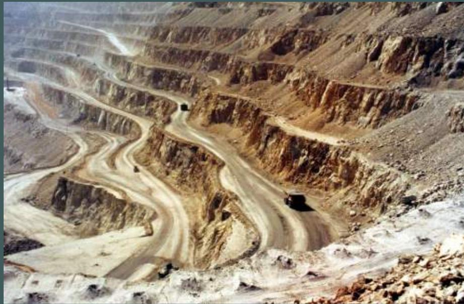
**Bench scale slopes at Chuquicamata are obviously structurally controlled**
