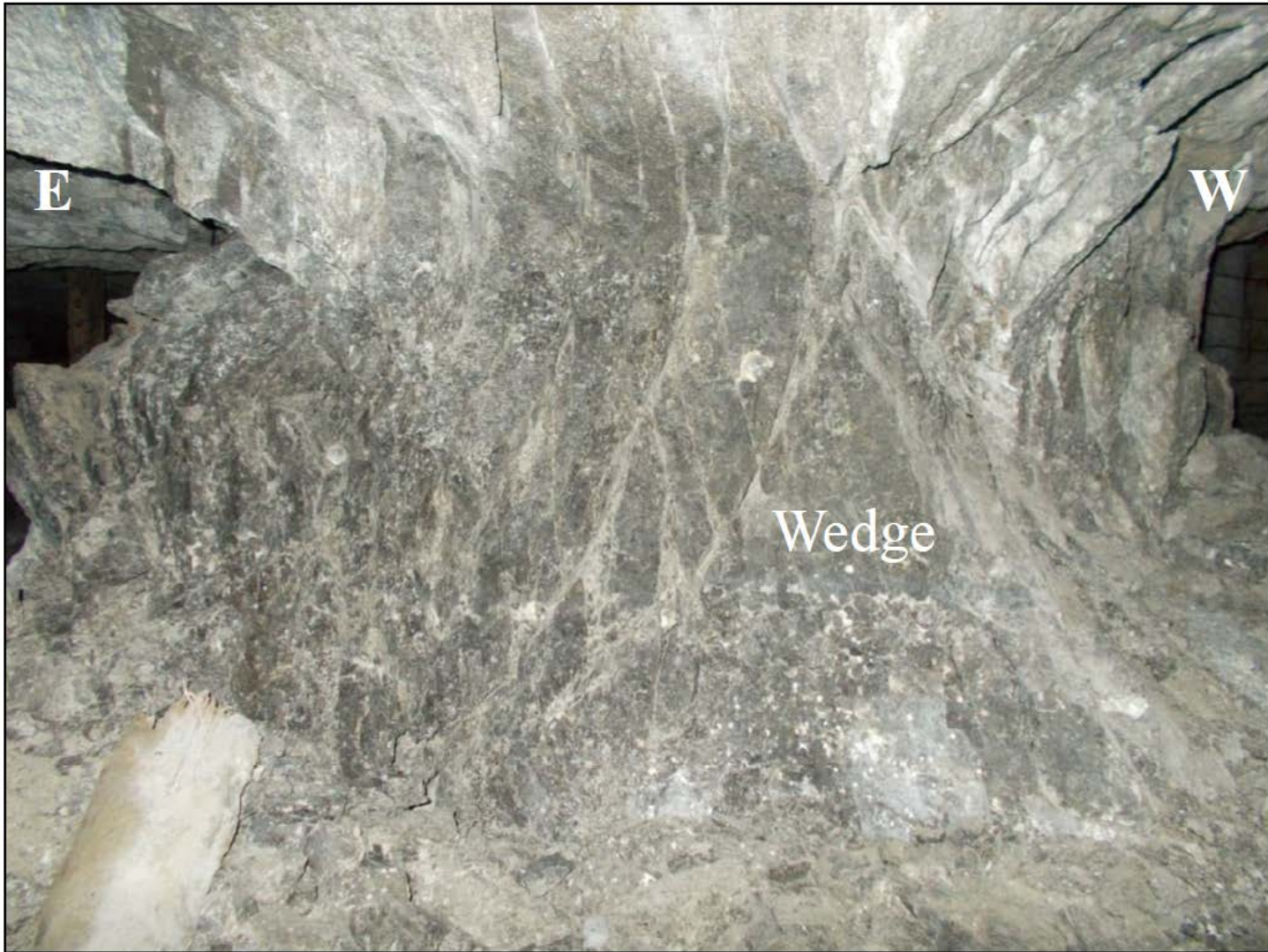
A crush pillar in a South African mine (M. du Plessis 2015)
