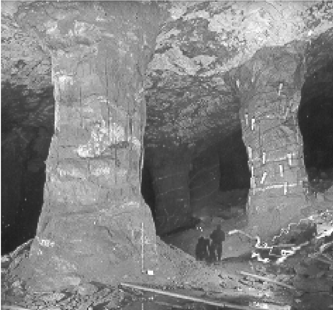
Spalling/slabbing in sandstone pillars
