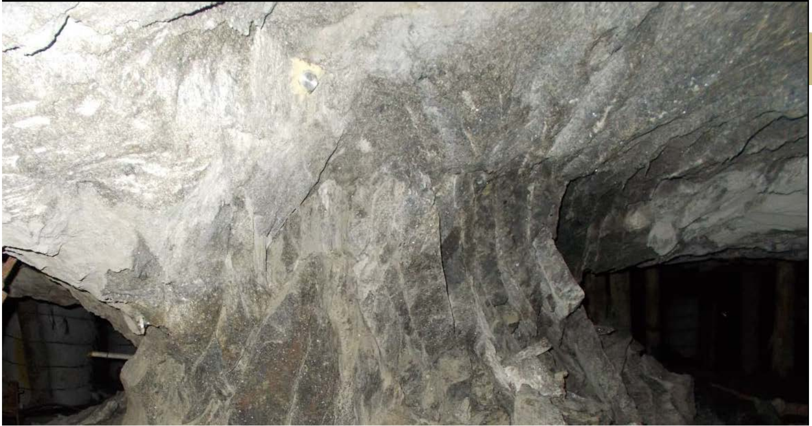
A crush pillar in a South African mine (M. du Plessis 2015)
