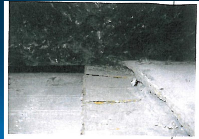
Single shielded TBM jammed in squeezing ground (Ramoni 2012)
