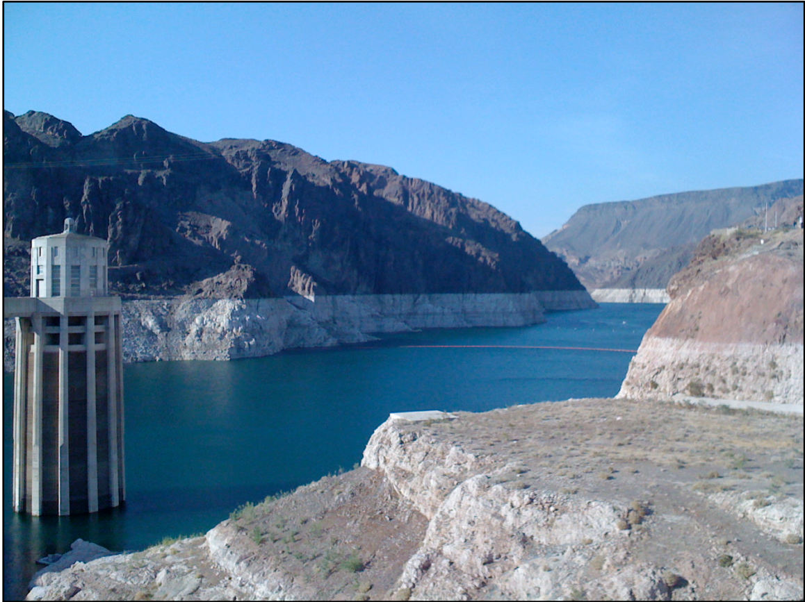
Here, a view from Hoover dam towards the lake.
