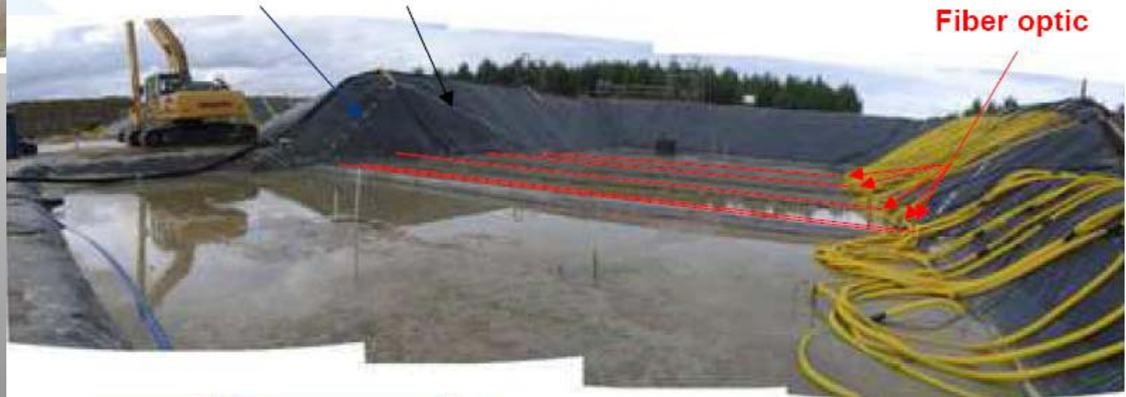
Downstream and upstream of the experimental dam
